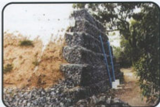
Six meter high MSE Test Embankment
