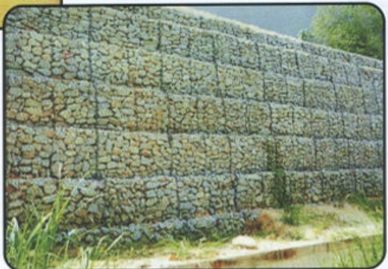
→ MSE Gabion Wall Seremban, Malaysia
