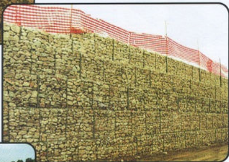
A 7.0m high 50 metre long MSE Gabion Wall being constructed
