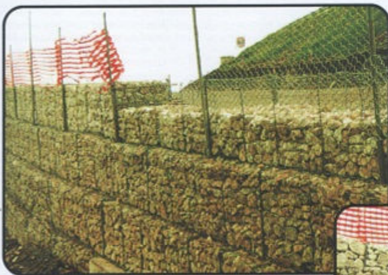
4.0m long facing gabions fabricated in horizontal mesh were used
