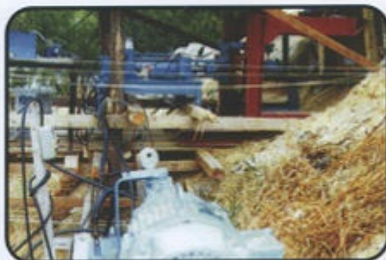
Field Pullout Test set up
