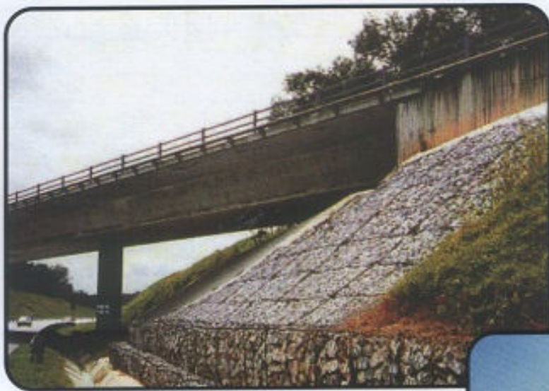
← Bridge Abutment Protection Tanjong Malim, Malaysia
