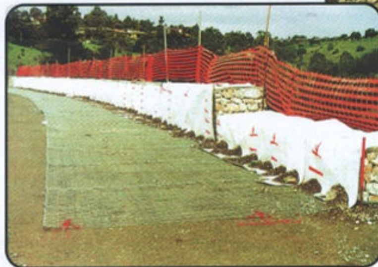
Adjacent 2.0m wide Panels were laced along their entire length and sandwiched between facing gabions prior to rockfilling
